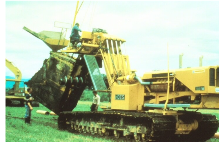
Lecture 12-2. Execution of drainage
